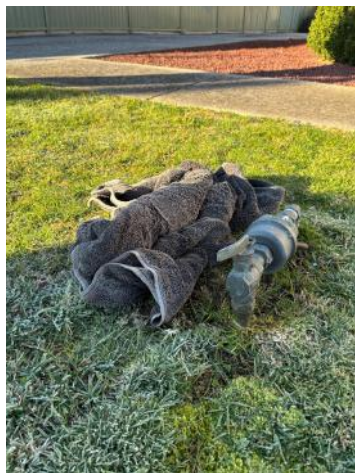
Covered traditional analog meter
